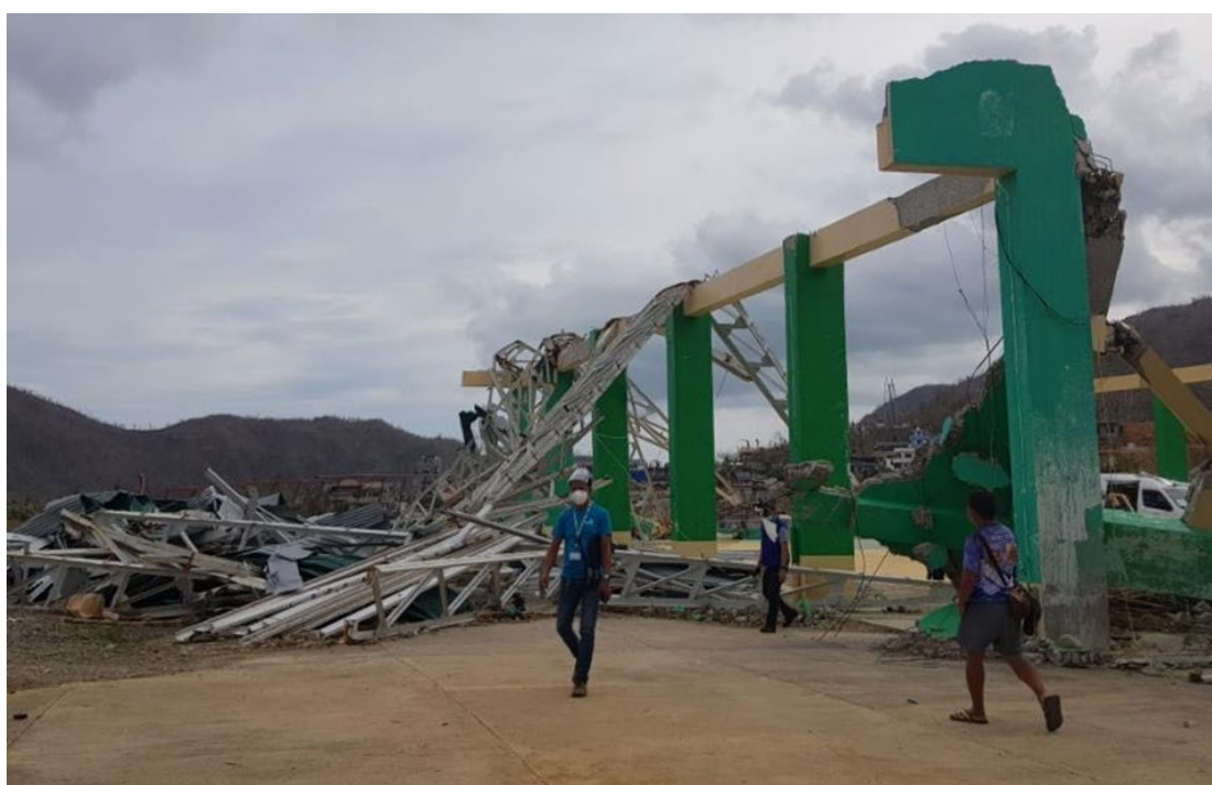
Catanduanes, 6 November 2020: Typhoon Goni tore off roofs and destroyed structures.
